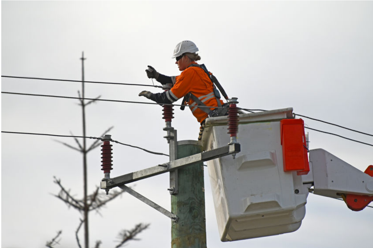
A worker performing high risk work on power lines.
