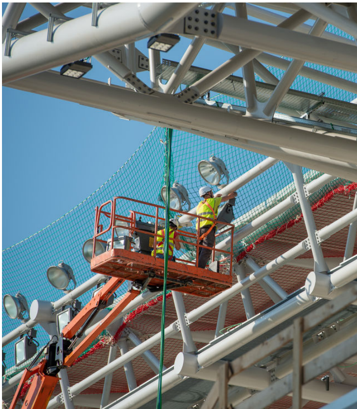
Workers undertaking high risk work using an Elevating Work Platform.
