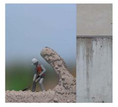
Also, man-made structures may introduce a large downward force on the soil below. For this reason, excavating near man-made structures requires special safety consideration.
