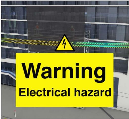
Permit conditions may require the hoarding to have the top edge extend above the work platform adjacent to the power line.
