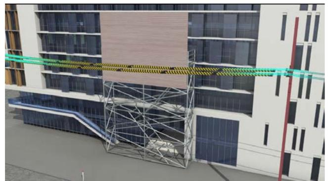
For example, where the safe clearance distance is 1.5 metres from a bare 415 volt line, the hoarding needs to extend 2.7 metres below the power line and continue to 2.4 metres above the power line (for more information on these distances, please contact the Office of the Technical Regulator on 8226 5500).
